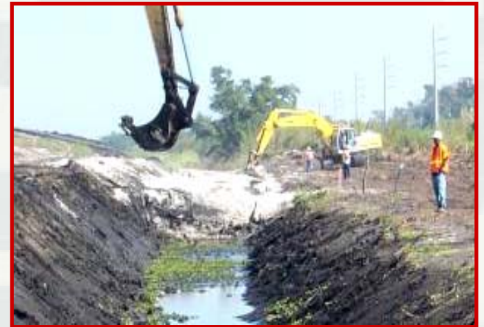
Tree removal and filling the landside ditch
