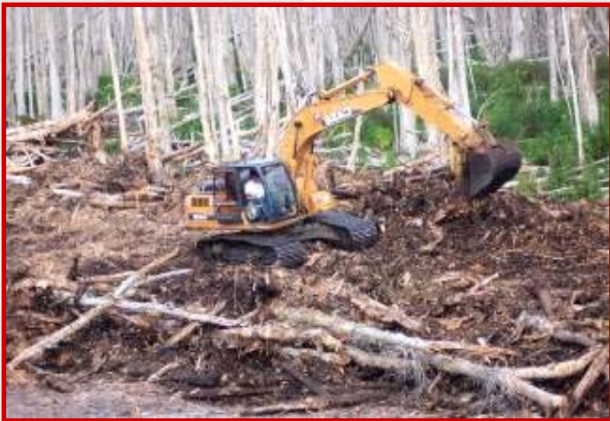
Tree removal and filling the landside ditch
